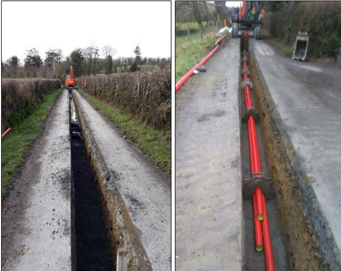
**Plates 2 & 3: Typical Trench Construction**
