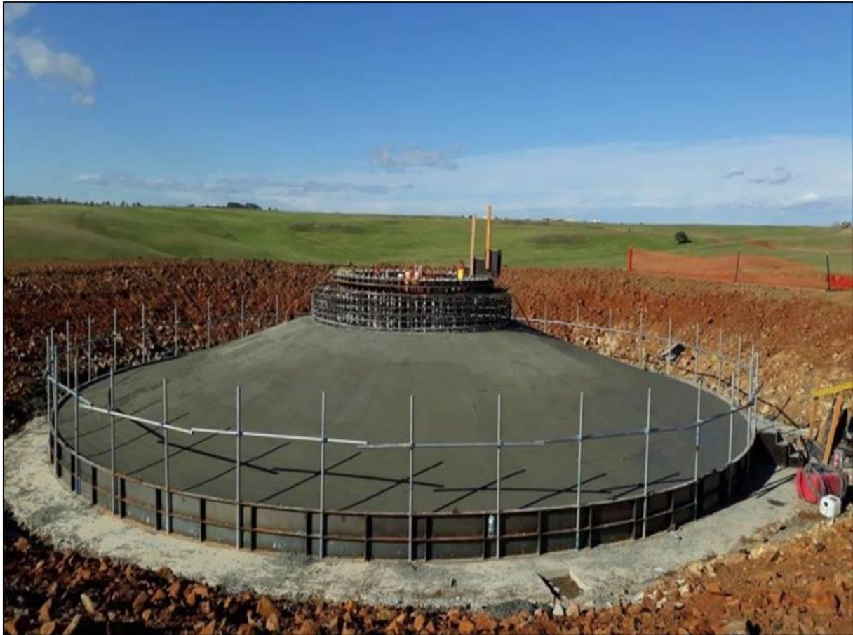
**Figure 3.5: Typical Turbine Foundation**
